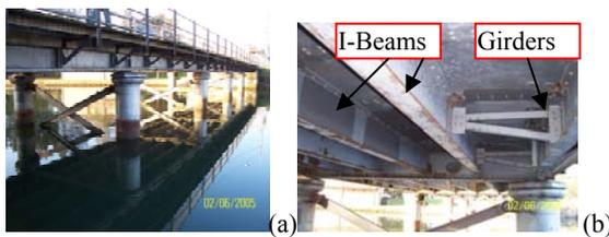
Figure 2 (a) An example bridge; (b) Part of the bridge structure
